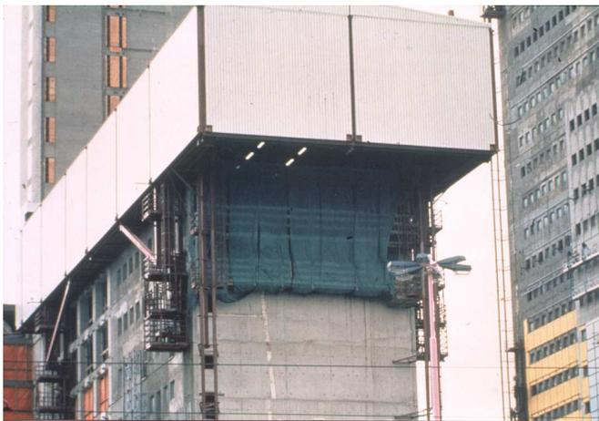
Fig. 1. Delftse Poort Mechanised Construction System
