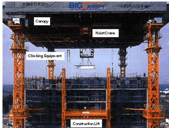
Fig. 2. Big Canopy automated construction system
