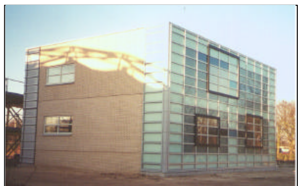
Figure 3. IFD building system trial module on the Eindhoven University of Technology campus.
