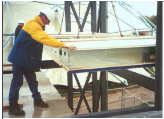
Figure 2. Assembling the floor panels.
