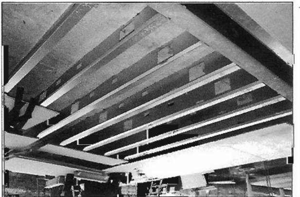
Figure 4 Van Dam floor system with one cold formed profile.
