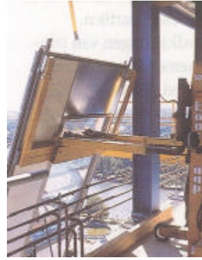
3. Wall panels are moved outside.
