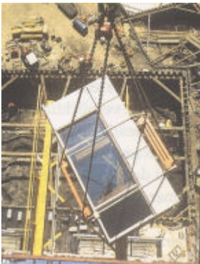
1. Wall panels are transported to the floor where they are required.
